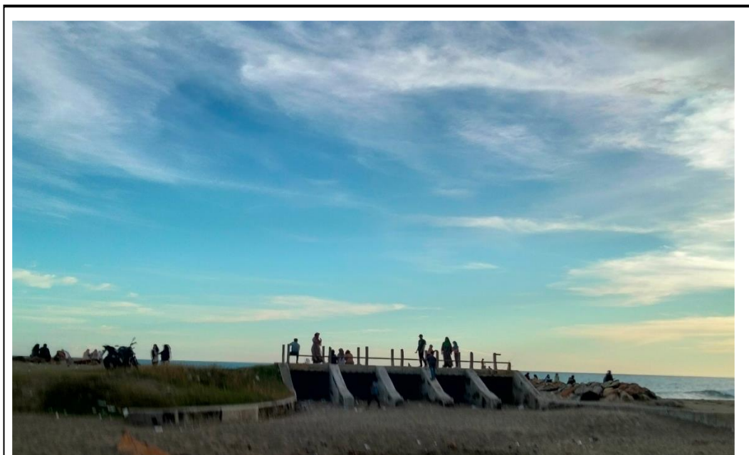
Gambar A.3.9 Floodgate
