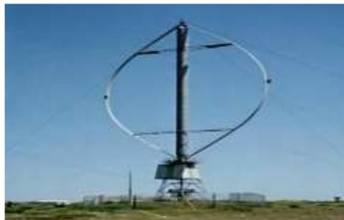
Gambar 2.2 Turbin Angin Sumbu *Vertical*
