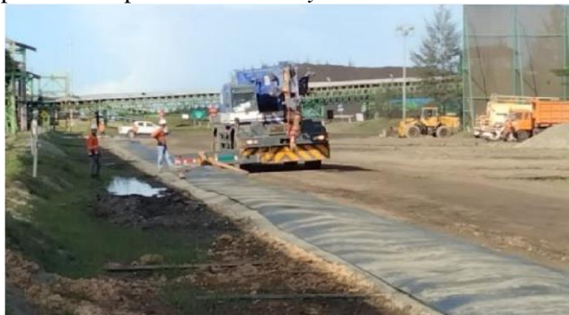
Gambar 3. Proses Lay UP Belt conpevor ,
