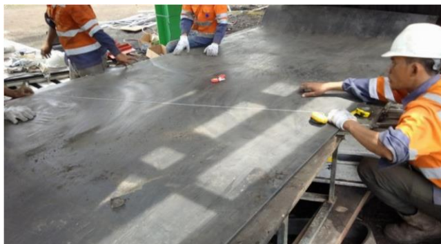
Gambar 4. Proses Pengukuran belt conveyor
