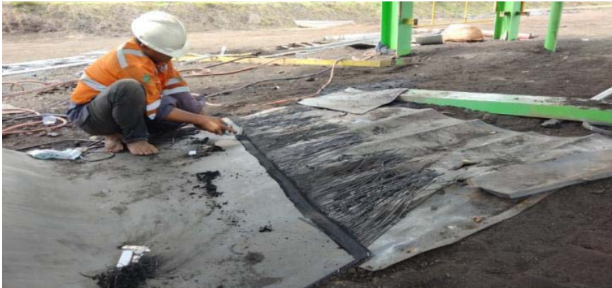
Gambar 2.5 Proses Pengerindaan Lapisan Belt Conveyor
