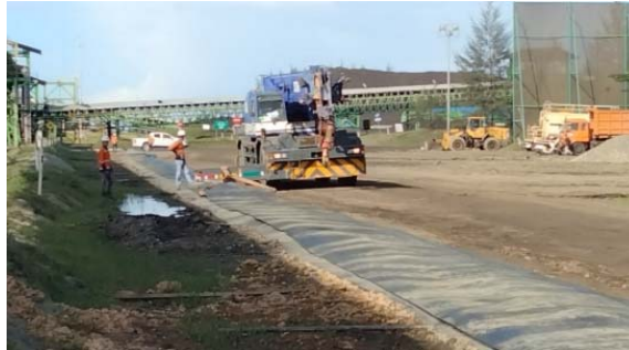
Gambar 2.1 Proses Lay Up Belt
