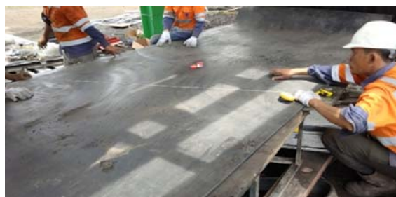
Gambar 2.2 Proses pengukuran Pemotongan Belt Conveyor
