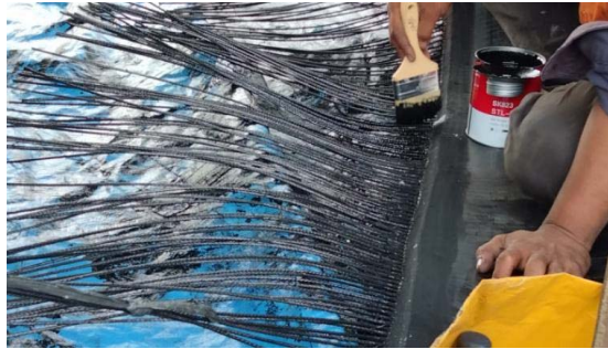
Gambar 2.6 Proses pengeleman belt conveyor
