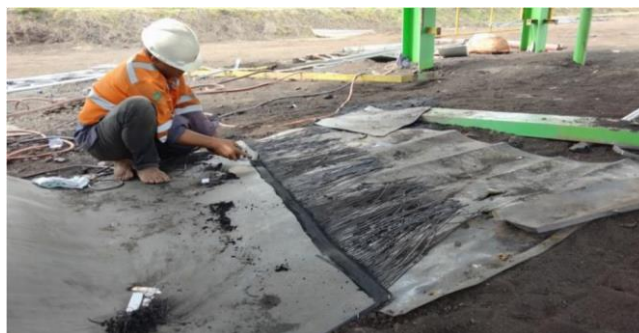
Gambar 7. Proses Pengerindaan Lapisan Belt Conveyor
