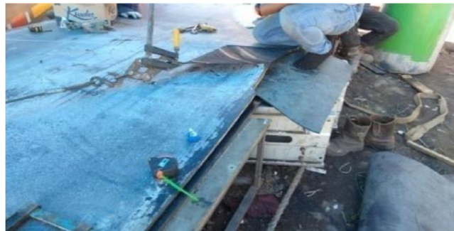
Gambar 6. Proses Pengupasan Belt Conveyor
